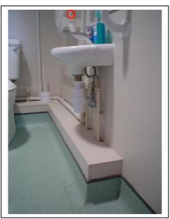
The boxing beneath the hand basin obstructs wheelchair user's wheels from positioning in front of the basin.
