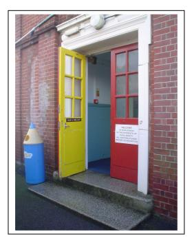
It does not have any handrails or highlight colour band for the nosings.
